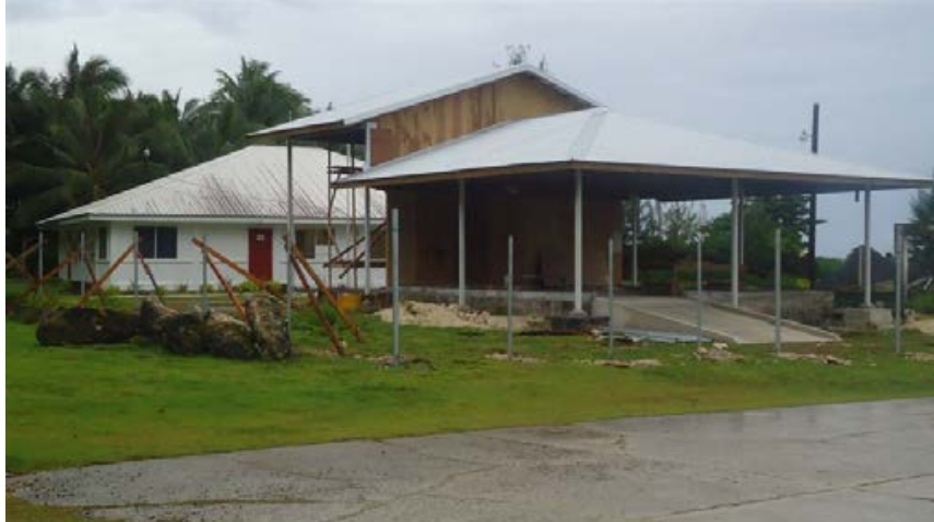
Construction of the storage fale (fuel and ice making) in the island of Ta'u (Photo:U.Faasili)
